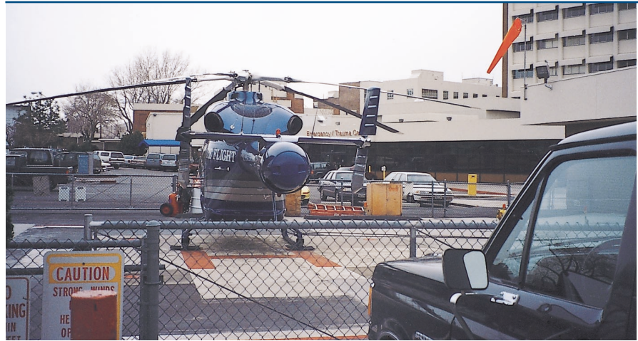
▲ Helicopter pad with fresh air intake
