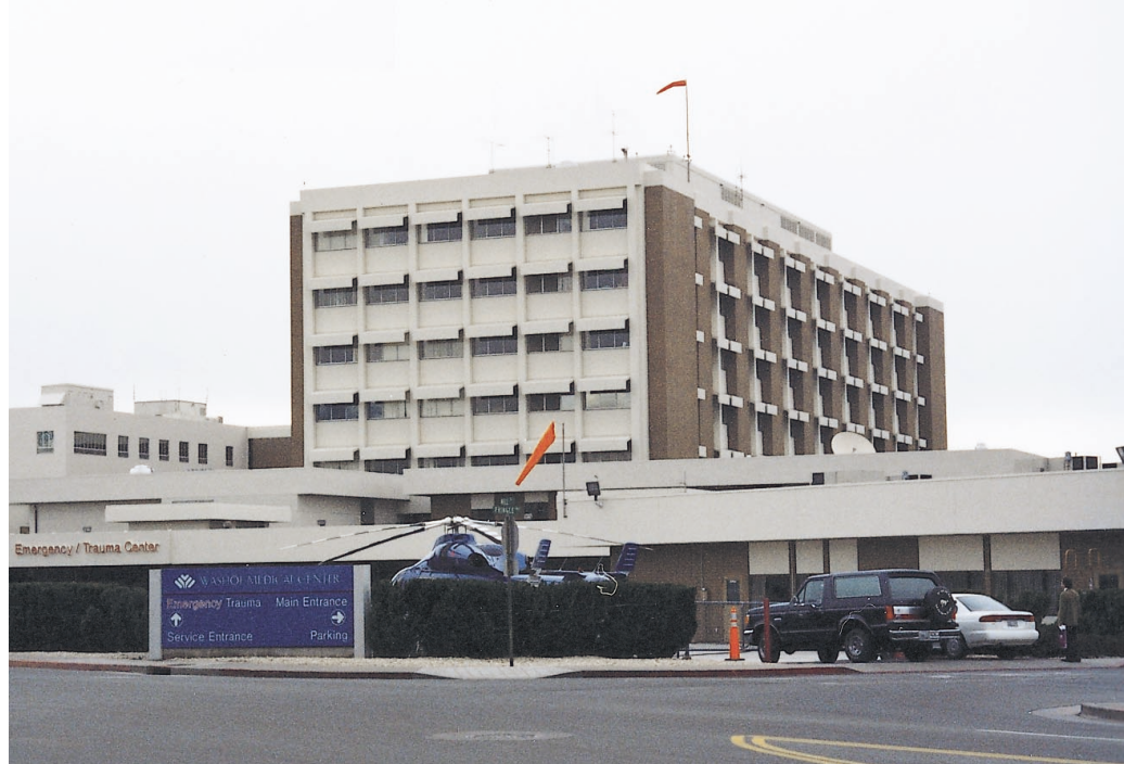
▲ Washoe Medical Center - Main Building
