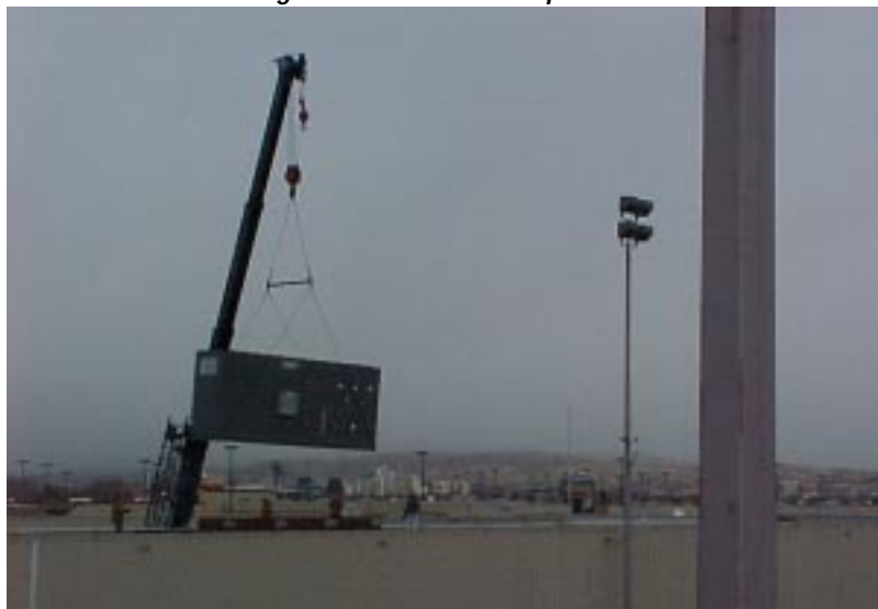
TMP-15000 unit being hoisted onto rooftop
